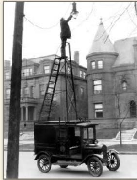
Electric Department changing s street lightbulb.
