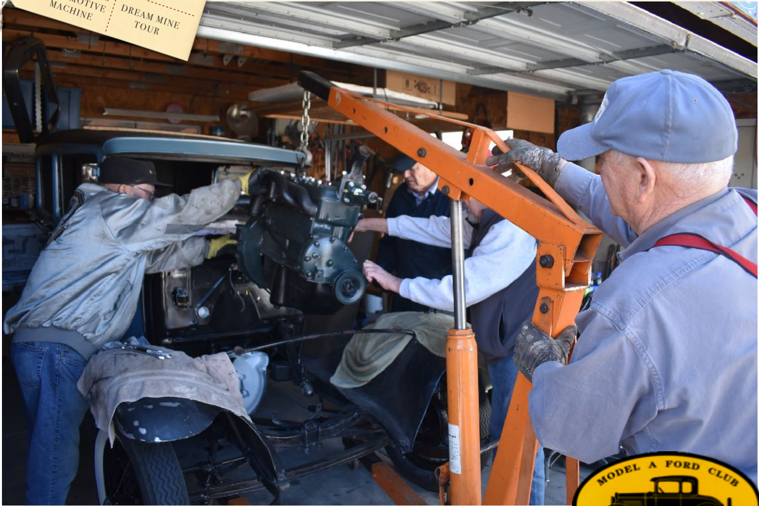
Garage Day, engine installation — Howard Eckstein photographer
