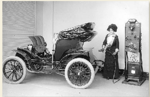
Figure 3: Electric Car Charging Station
