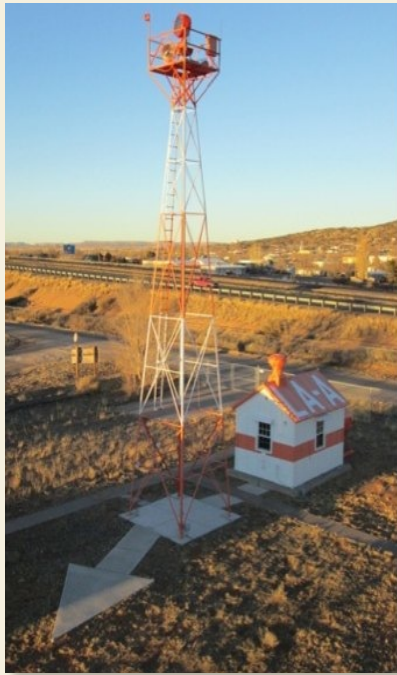
Restored beacon tower and maintenance/gas shed. Located at the Grants-Milian Historic Aviation museum.
